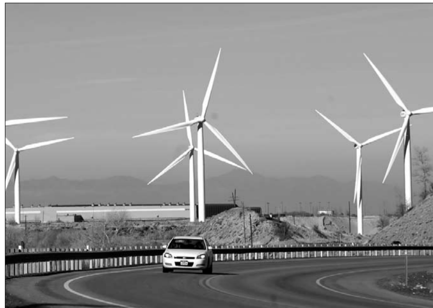
A car makes its way up U.S. Highway 6 past several 2.1 mega watt wind powered turbines owned at the mouth of Spanish Fork Canyon in Spanish Fork, Utah. Wind and solar power could produce 40 percent of the world's electricity by 2050 if government subsidies are secured for the next two decades, scientists said on Wednesday.
