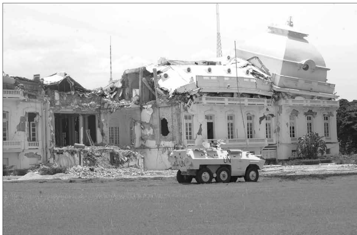
STILL IN RUINS: The Presidential Palace in Haiti's capital, Port-au-Prince, on May 12. Five months after a devastating earthquake hit Haiti, there have been no signs of reconstruction of the palace, making it emblematic of the country's stalled rebuilding process. THONY BELIZAIRE/AFP/GETTY IMAGES
